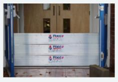
**Figure 1** Demountable barrier for external door 1 donated by www.floodtec.co.uk
