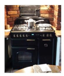
**Figure 3** Range in tanked alcove has its own flood barrier
