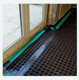
**Figure 5** Channels and membranes with sumps and pumps to remove water
