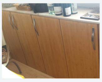
Figure 8 The bamboo kitchen units survived the flood intact (despite being submerged for 17 hours)
