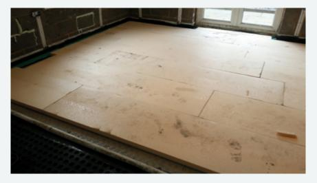
Figure 6 Closed cell (waterproof) insulation on the floor
