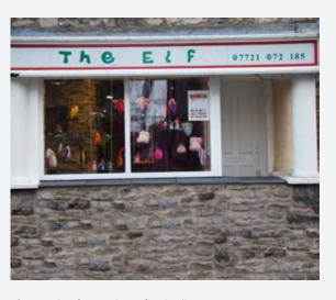
**Figure 3** Shop front, with new flood wall to deflect bow waves' caused by passing vehicles
