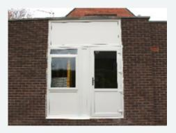
**Figure 3** Flood resistant side door donated by www.floodsmartsystems.co.uk
