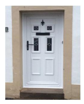
**Figure 5** A flood-resistant door has been installed, which allows additional time for moving items before the water has to be let in. Installation by Floodsafe Projects Ltd (www.floodsafeprojects.co.uk)
