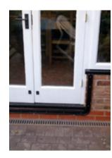
**Figure 1** Non-standard doorway with unobtrusive barrier fittings
