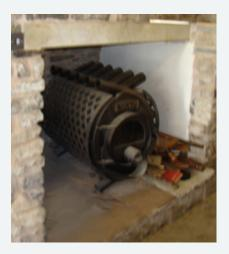
**Figure 5** Wood-burning stove, housed within body of stone staircase (German 18kw design)
