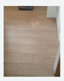
**Figure 7** Finished with 'Aquastep' removable plastic flooring and skirtings
