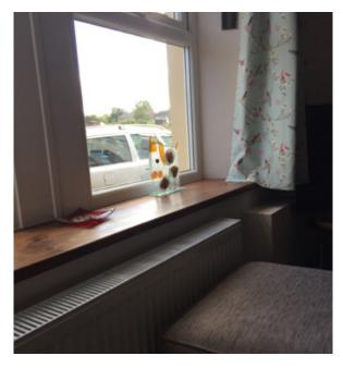
**Figure 2** The window sills are made of hardwood (instead of the usual easily-damaged softwood)
