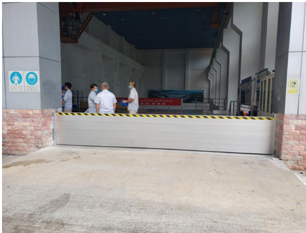
Friiva™ Door gate flood protection single span with mounting post on the side
