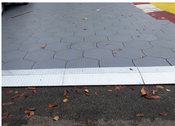
Steel Ramp for Heavy Vehicles
