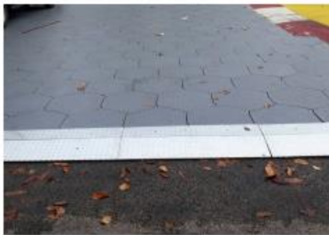
Steel Ramp for Heavy Vehicles
