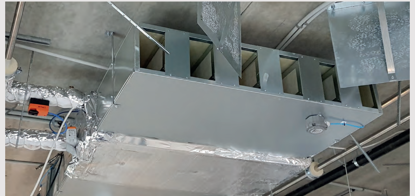
Fan Coils mounted over the ceiling
