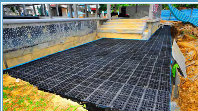
FlexaTank Retention System installed at a residential house
