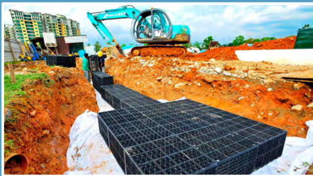
FlexaTank Infiltration System installed at a park
