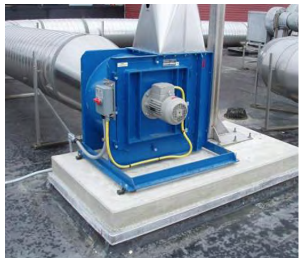
Fan placed on the roof.
